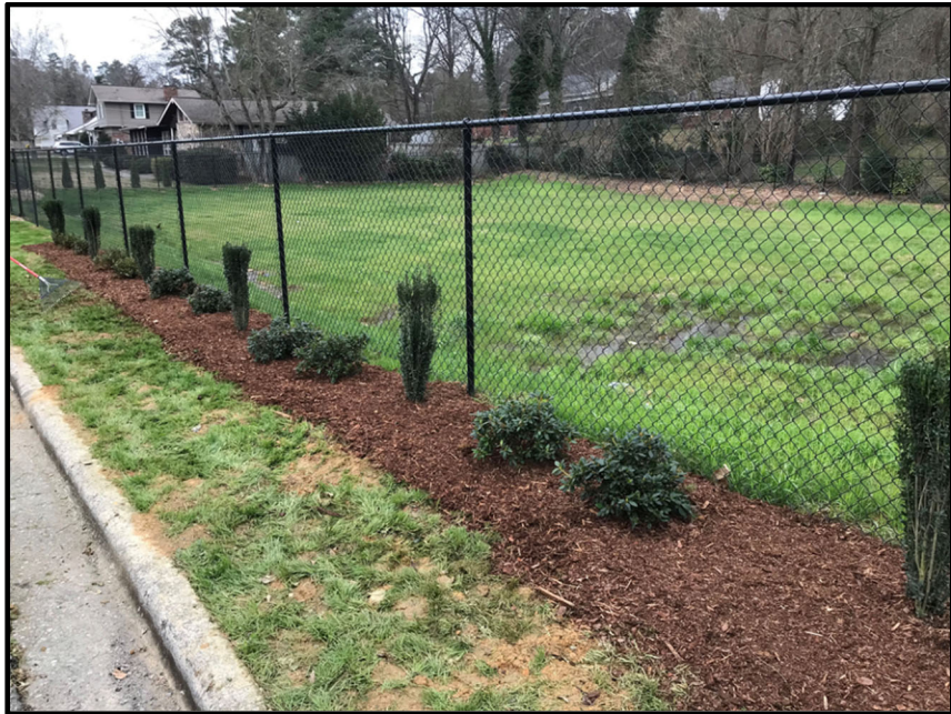
Brookwood Drive Regional Flood Storage and Stormwater Detention Project Completed
