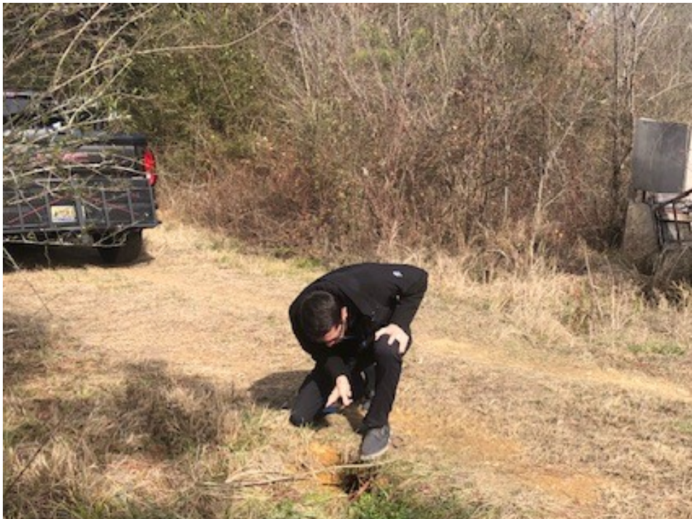
Existing pipe culvert crossing that may require replacement. Looking East
